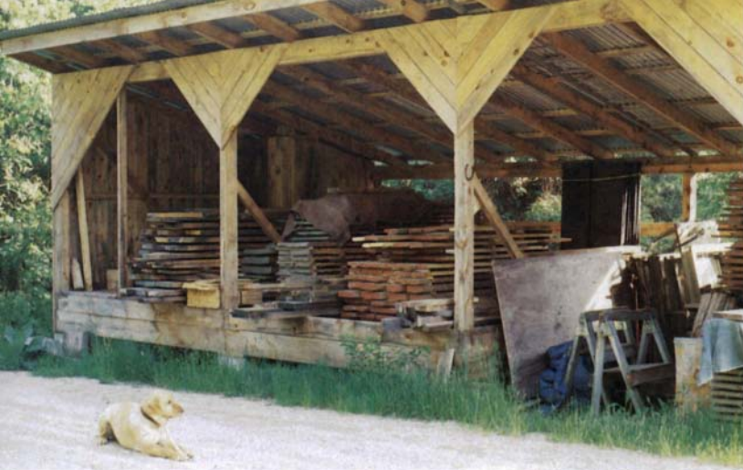
Rhode Island woodworker Geoff Warner's drying shed has a large overhang to protect lumber against rain. Although not critical, lumber sheds should be oriented to be open to the north, with the southern exposure covered to prevent losses from rapid drying.
