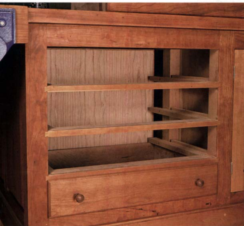
Drawers are supported by a runner that is mortised and tenoned to the drawer divider and then screwed to the center stile. A drawer guide screwed to the runner keeps the drawer aligned for easy closing.
